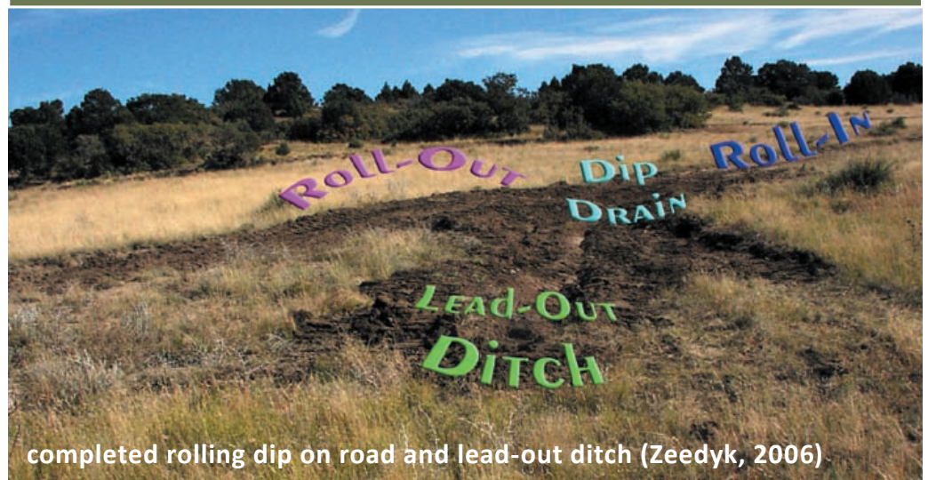
Rolling Dip schematic (Zeedyk, 2006)
