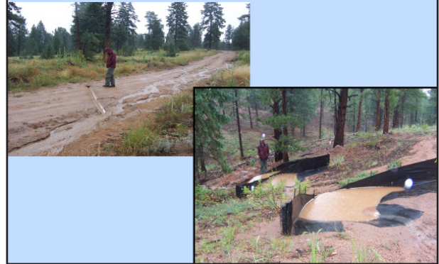
Figure 24. Unpaved roads are often the dominant source of anthropogenic sediment in forested watersheds.
