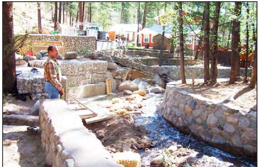
Figure 3. Following multiple attempts at bank stabilization to protect encroaching urban infrastructure, the Rio Ruidoso has been reduced to a concrete canal with loss of all natural function except water transport.
