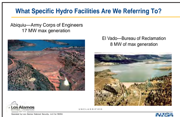
Figure 1. Hydro stations owned and operated by Los Alamos County Department of Public Utilities
