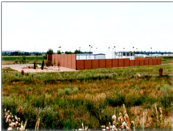
Figure 3. Completed Cloud Computing Facility in Longmont, Colorado
