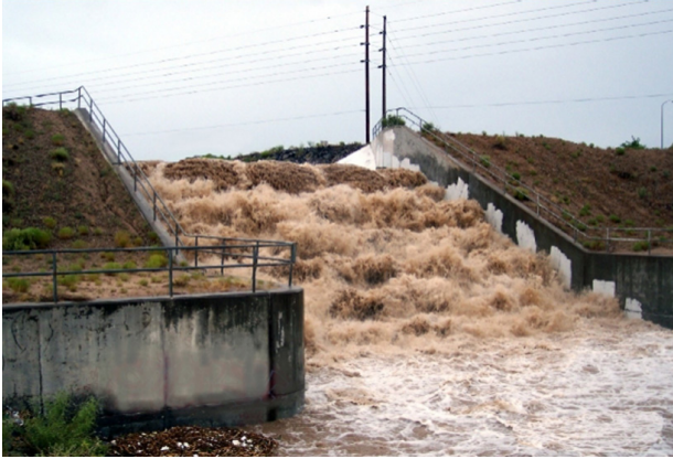
Figure 1. South Diversion Channel Drop Structure
