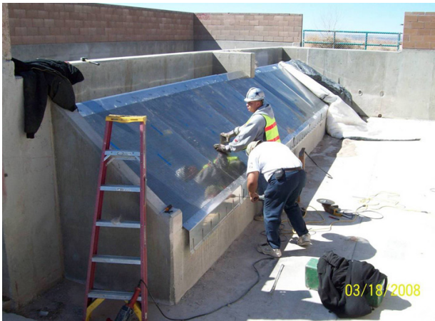
Figure 16. Coanda Screen Installation over New Clean Water Gallery
