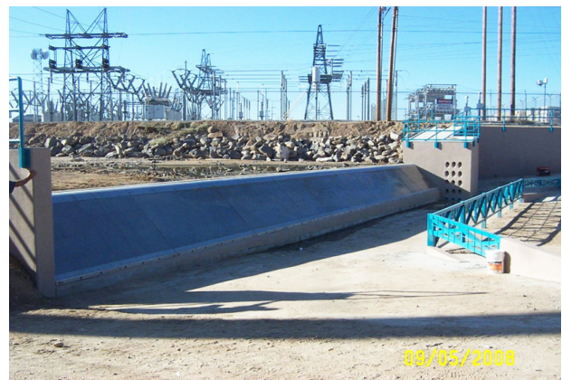
Figure 18. Vineyard Arroyo SWQF Complete
