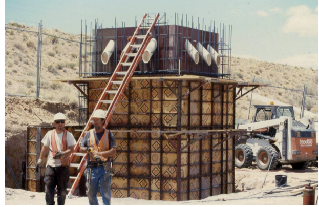
Figure 9. Inclined Port Spillway Tower at South Baca Dam
