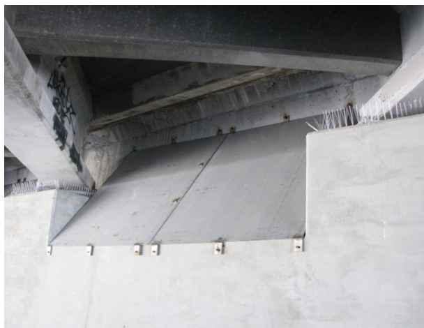
Figure 23. North Diversion Channel, Indian School Bridge Avian Control Project - Bird Spikes and Spiders
