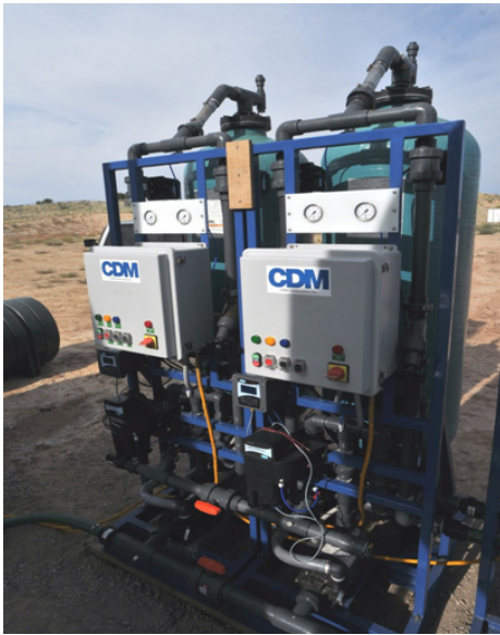
Figure 4. Pre-filter System (sand & anthracite)
