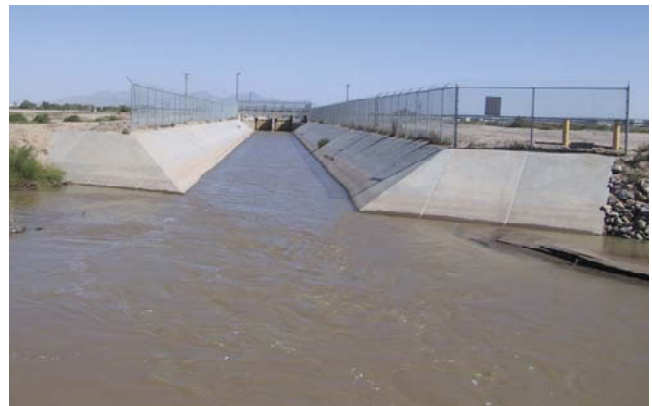
Figure 4. American Canal Extension
