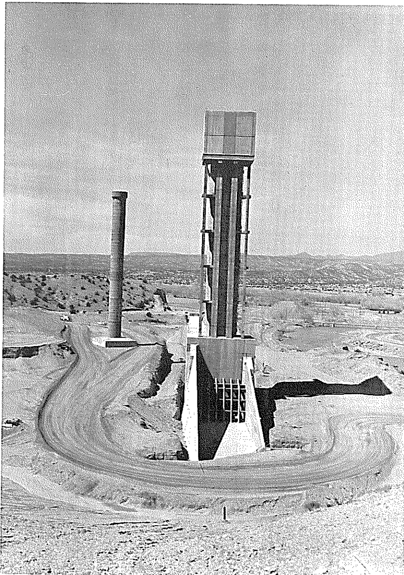
View of the intake structure of the outlet works. If you look very closely - you can see a man standing next to the trash rack on the concrete floor of the intake.
