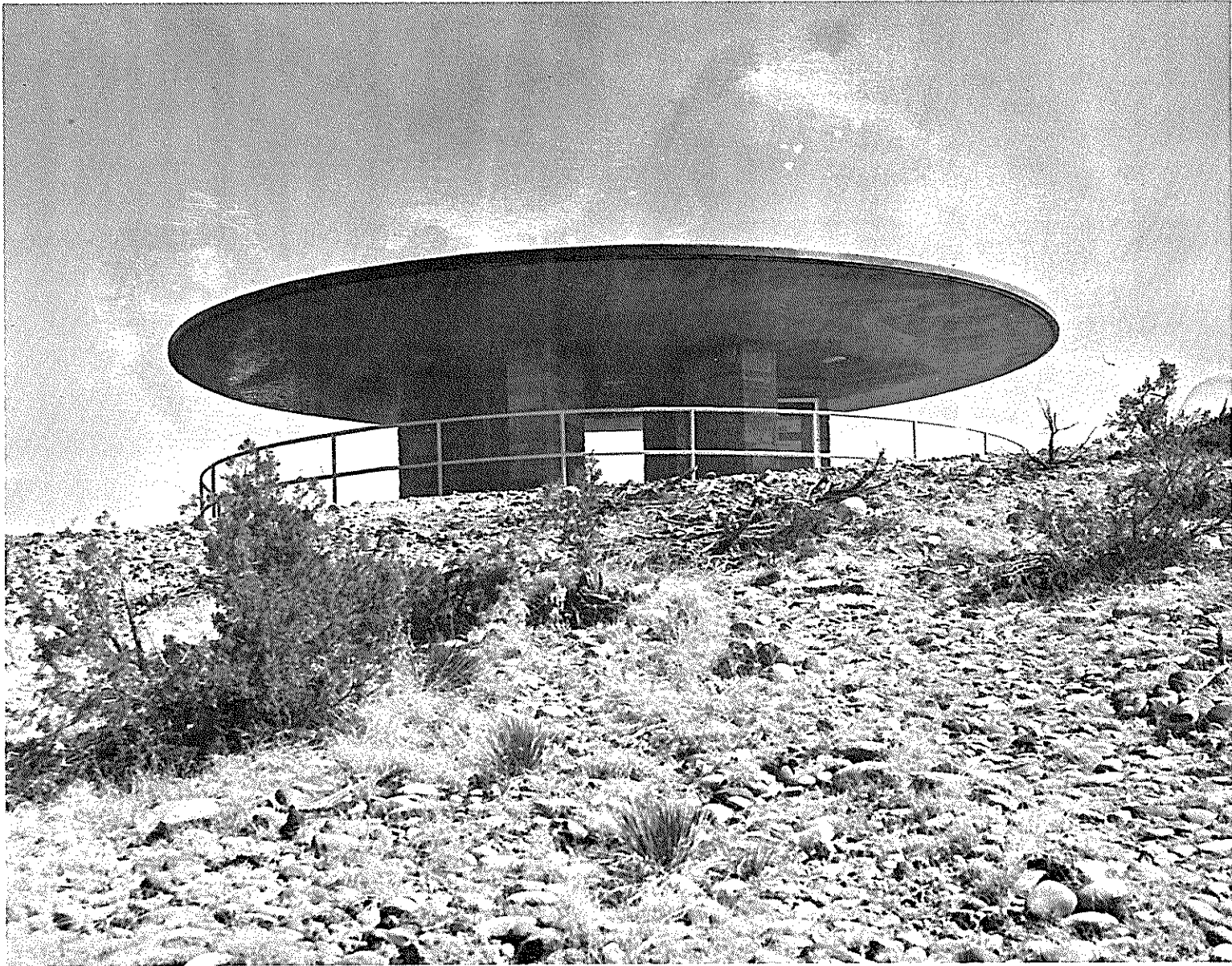
Close-up view of the recently completed Cochiti Overlook.
