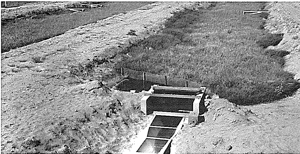
Effluent channel in Salt River bed west of Phoenix, carrying a flow of about 50 mgd (about 80 cfs).
