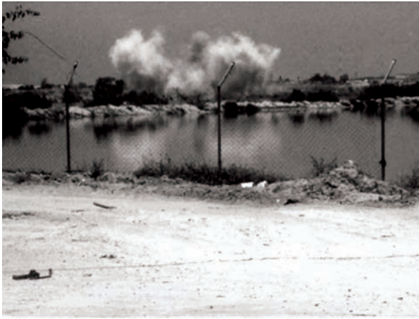
Figure 1. North Wastewater Treatment plant in Beit Lahiya, Gaza Strip under bombardment with dust cloud billowing up.
