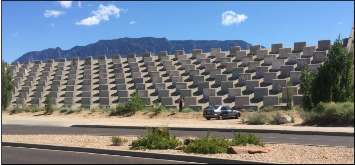
Figure 11. Photograph of the John B. Robert detention dam, a 65-ft (20 m) tall earthen dry dam owned and operated by the Albuquerque Metropolitan Arroyo Flood Control Authority (AMAFCA) (photo by the author).
