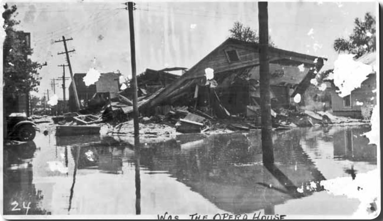
This photo from the San Marcial flood of 1929 is an example of unintended consequences of other actions in the Rio Grande Valley. Overgrazing and clear cutting in the headwaters of the Rio Grande and heavy diversions of irrigation water in the San Luis Valley caused increased erosion and decreased flow. The result was river bed sediment raising the river level above the land surface (14 feet above the streets of San Marcial, for example). Loss of vegetation caused the river level to spike rapidly and made overtopping of the levees, followed by complete inundation, inevitable. (Photo courtesy of Socorro County Historical Society)
