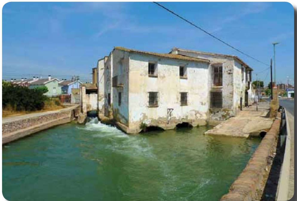
Valencia irrigators receive water after human use, community use, and industrial use, but physical systems are in place to ensure that irrigators have top priority in times of water scarcity. Note two canals allowing water to turn a water mill inside the building in the picture and a third canal to the left of the structure for by-passing the mills. (Photo courtesy of Luis Pablo Martinez)
