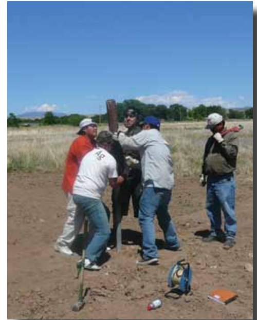
Undergraduate students and David Archuleta (far right) install a groundwater monitoring well at the Sustainable Agriculture Science Center at Alcalde, one of Dr. Fernald's research sites.
