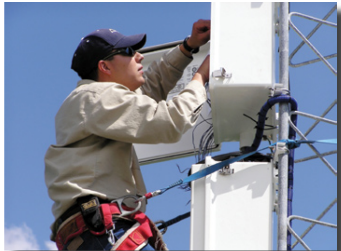
Jimmy wires the sensors to the data logger.
