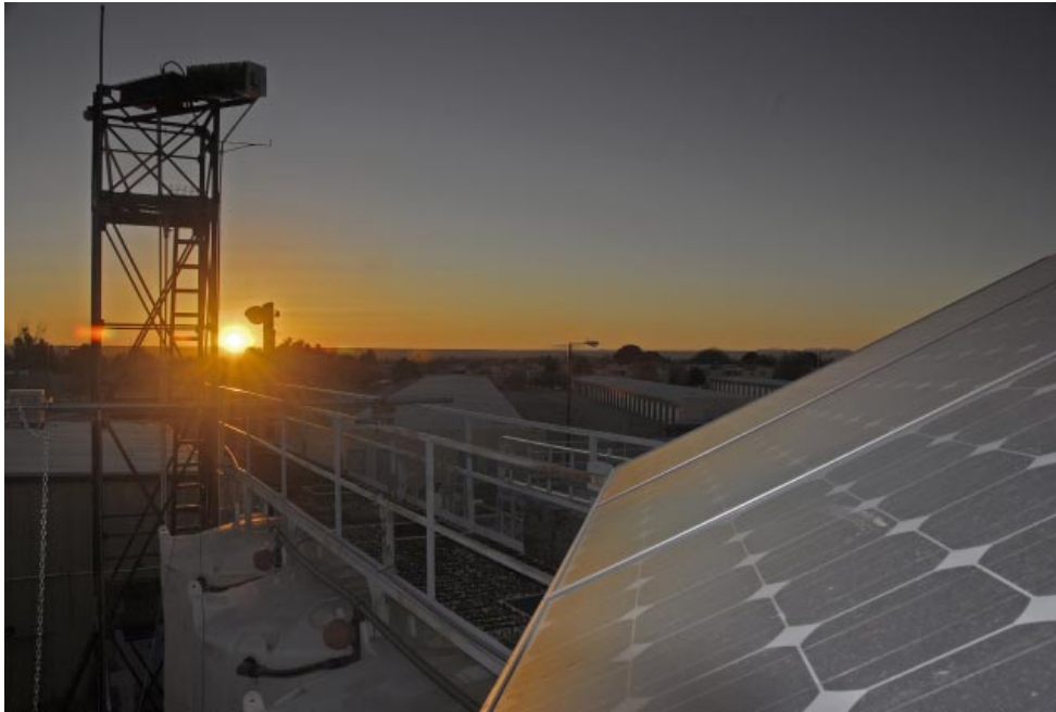
A photovoltaic module (in the foreground) captures the last rays of the sun to produce electricity, which is used to drive this desalination process (in the background). (Photo by N. Khandan)
