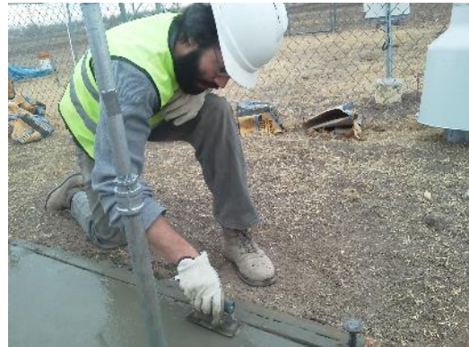
Figure 8. Garrett Gibson installing Pluvio rain gauge at Leyendecker
