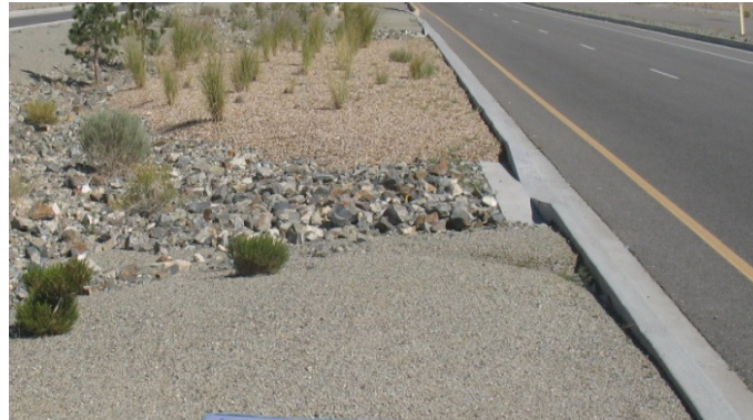
Figure 16: Green street with cube cuts and native vegetation. University Blvd at Mesa Del Sol, Albuquerque.
