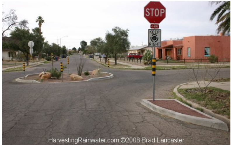
Figure 9: Traffic calming round-about that also harvests street runoff. Source: Brad Lancaster, www.harvestingrainwater.com
