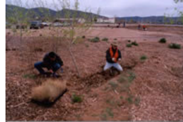
Figure 18: Juan Tabo demonstration site, where swales were installed with native vegetation to control runoff along Interstate 40 in Albuquerque. Source: www.ciudadswcd.org
