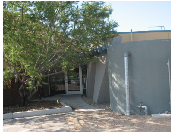
Figure 13: Cistern at SCAFCA offices, Rio Rancho, NM.
