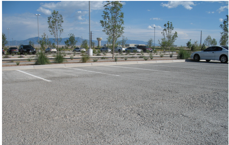
Figure 21: Porous pavement. Mesa del Sol, Albuquerque, NM.
