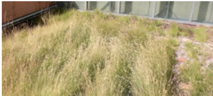
Figure 22: A “living roof” at the School of Architecture and Planning, University of New Mexico. The term “living roof” is used instead to more accurately reflect the native plant pallet used. This roof was designed to be irrigated with either potable or harvested water, and is currently being monitored to quantify benefits and hydrologic activity.
