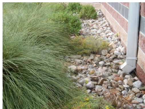
Figure 19: An infiltration planter. Downspout drains to vegetation area at Pavilions Shopping Plaza, Albuquerque, NM.
