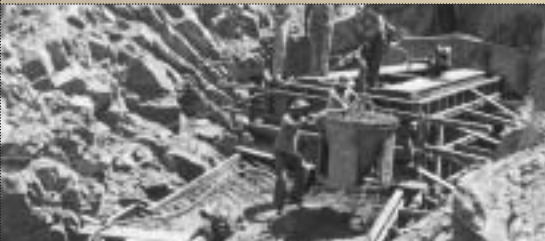
IMAGE: Workers place concrete for structure at inlet portal of San Vicente Tunnel.
