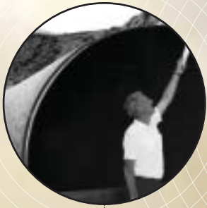
IMAGE: Pipeline 4: 96-inch-diameter welded steel pipe
