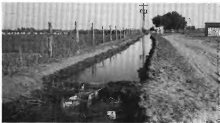
A. PARSHALL FLUME USED IN MEASURING DISCHARGES OF LARGE WELLS.
