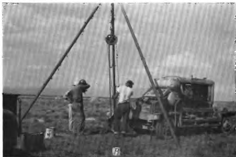
B. PULLING WELL PIPE AFTER COMPLETION OF TEST. JETTING OBSERVATION WELLS.
