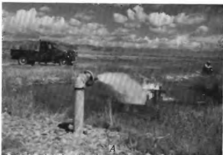
A. WELL 43-8 31bc2 DISCHARGING AT THE RATE OF ABOUT 580 GALLONS A MINUTE.
