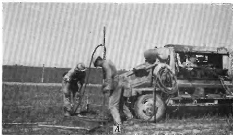
A. PUTTING DOWN OBSERVATION WELL BY MEANS OF COMPRESSED AIR.
