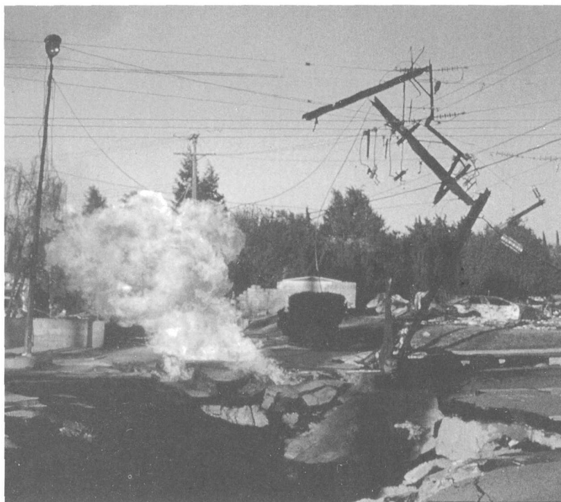
A ruptured gas main along Balboa Boulevard in Granada Hills caused this fire. Several homes in the area burned down, but, because there was no wind, most fires were easily contained.
