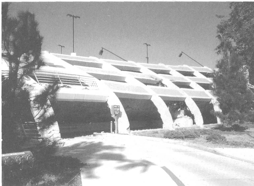
Strong shaking from the Northridge earthquake collapsed this parking structure on the campus of the California State University at Northridge. Because the earthquake occurred at 4:30 a.m., no people were in the structure.
