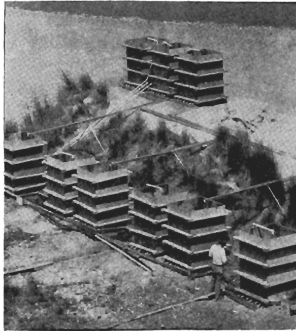
Figure 2. Pilot scale field intermittent sand filters at the Logan Sewage Lagoons.
