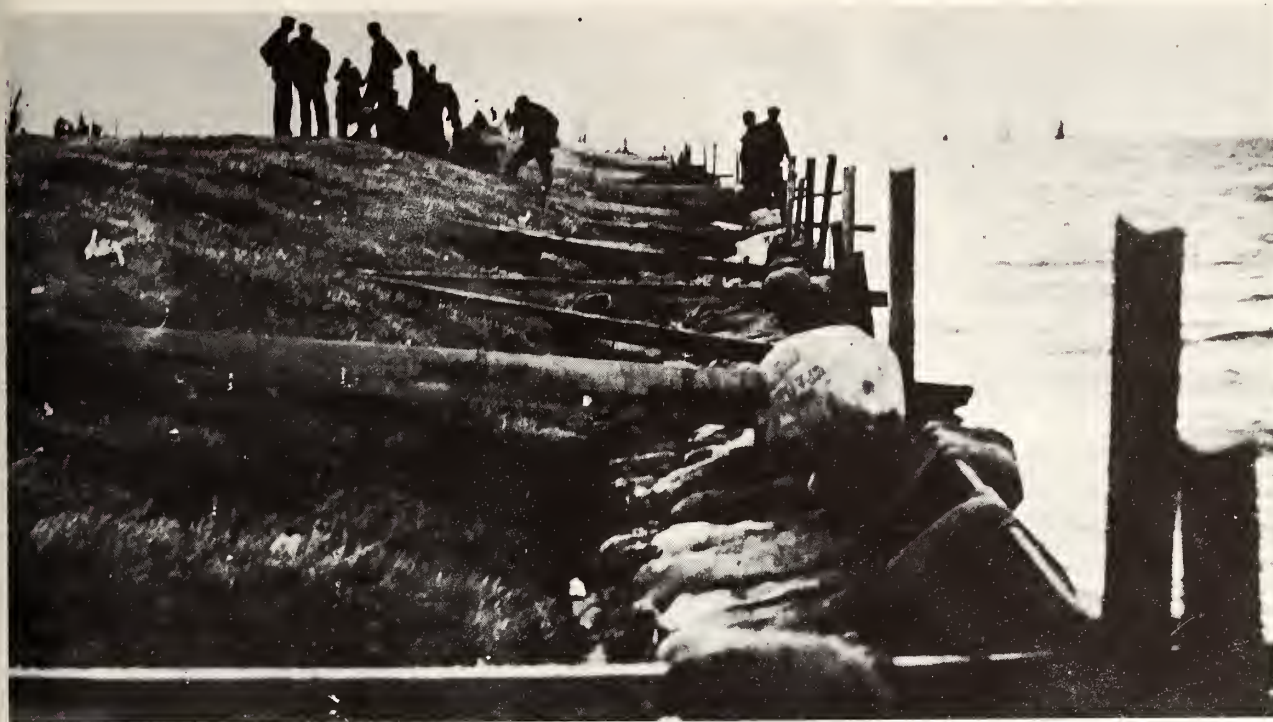
FIGURE 118.—Protecting Mississippi levee against wave wash during 1937 high water. (Large waves lashing the earth sides of the levees wash away the earth and are a serious menace to the levees. Here a crew of high water fighters has hastily constructed a board fence backed up by sand bags to protect the levee.)
