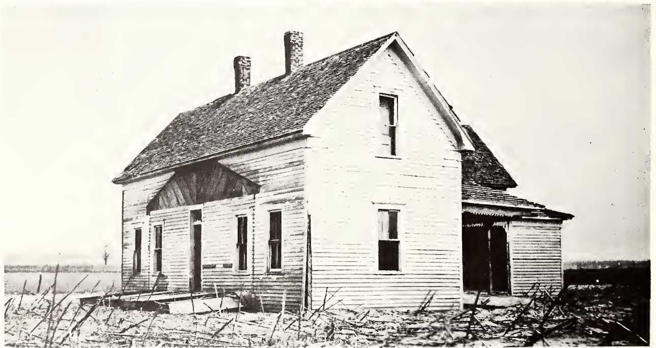
FIGURE 81.—Birds Point-New Madrid floodway after it had been opened and used in 1937 to alleviate flooding at Cairo. Top view: Wrecked school building. Middle view: Farm machinery battered and mangled out of shape. Bottom view: Dwelling floated from its foundation and stranded in corn field over a mile away when flood receded.
