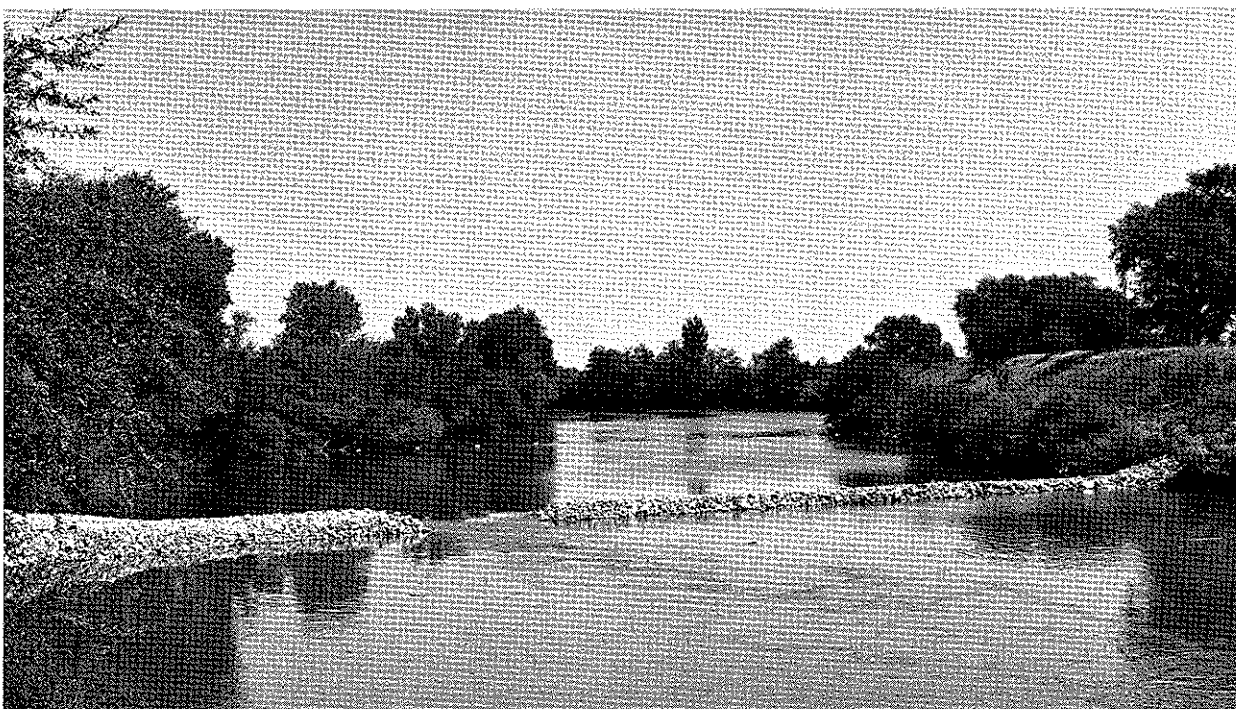
Sutter Slough rock barrier. In late summer, 1976, the Department of Water Resources installed an emergency rock barrier in Sutter Slough to force more of the Sacramento River's flow past the Delta cross-channel at Walnut Grove, where water could be diverted to the San Joaquin Delta.
