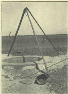
Fig. 13.—Well pit with concrete curbing extending to water level.
