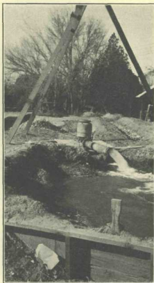
Pumping plant on the farm of the New Mexico Agricultural Experiment Station, State College, N. M. The discharge is 1625 gallons a minute from a 12-inch turbine pump installed in a 16-inch well.
