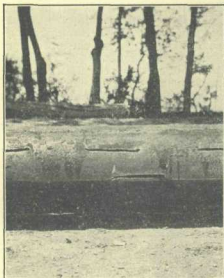
Fig. 9.—Perforated 12-inch casing used in New Mexico Experiment Station Horticultural Farm Well No. 3, drilled in 1935. Perforations are \frac{1}{8} inch by 8 inches, and were made with an acetylene torch.
