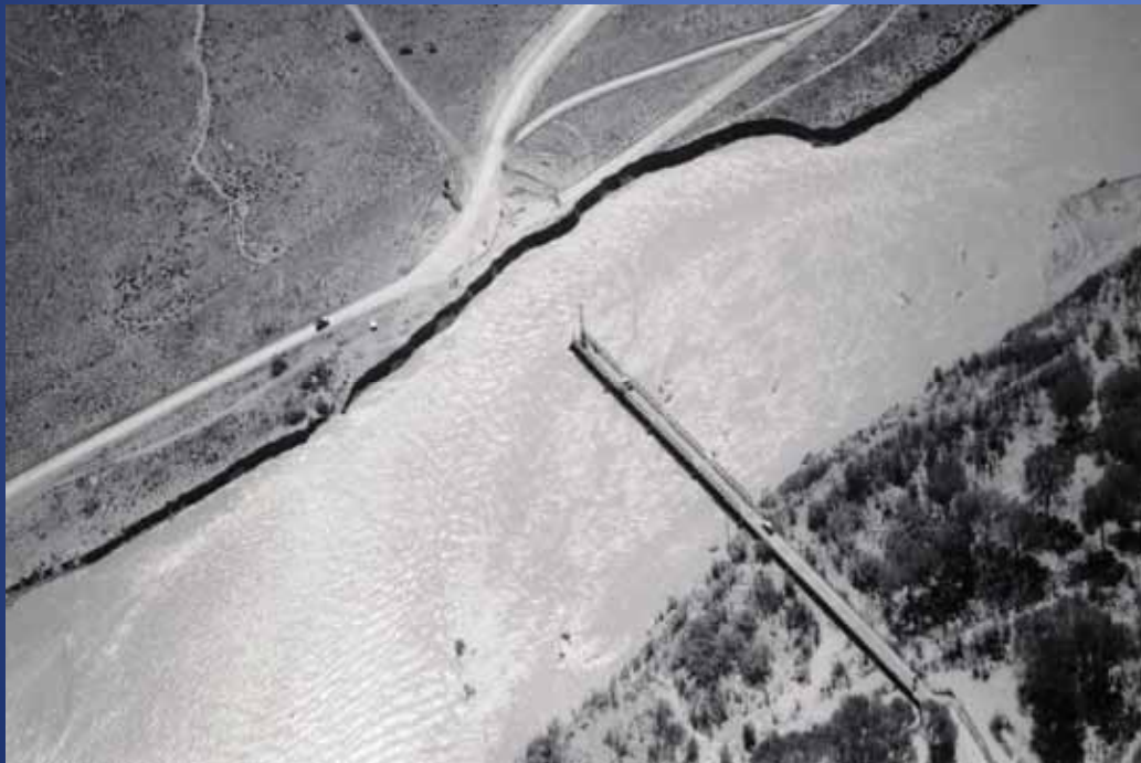
1941 Belen Bridge Washout
