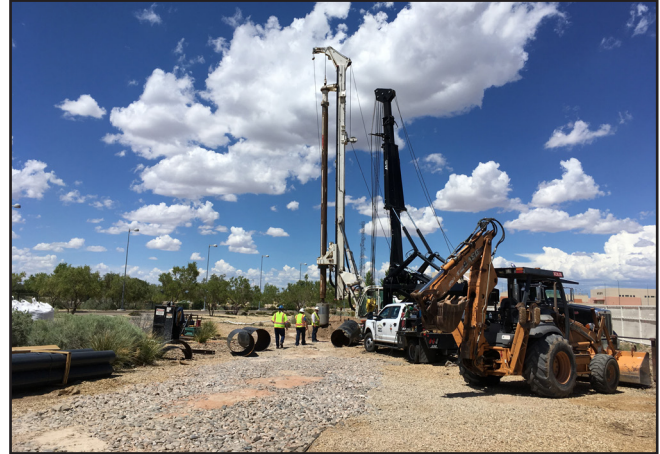
Figure 11. Vadose zone well drilling.
