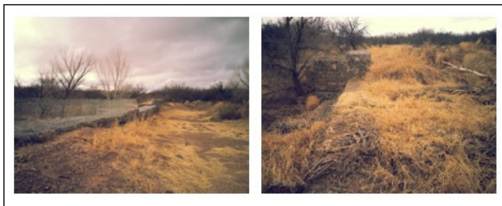
Figure 6. Gabion-style rock structures.
