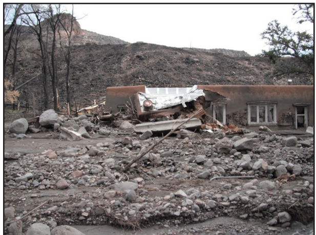
Figure 7. Property damage caused by post-fire flooding after the Las Conchas fire.
