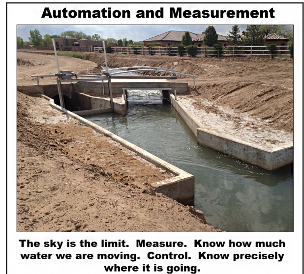
Figure 15. Benefits of flume measurement.
