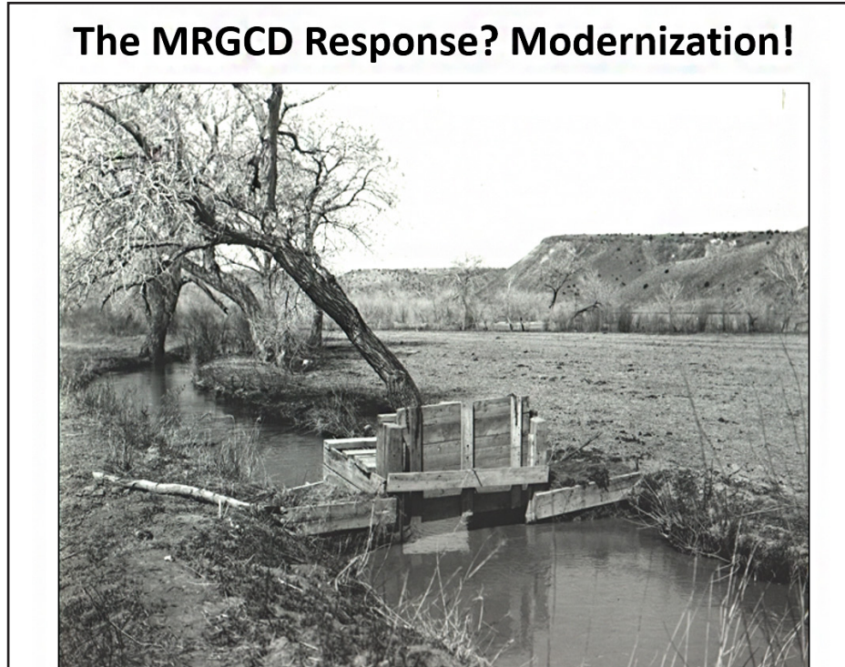
Figure 10. Middle Rio Grande Conservation District check structure at Algodones.
