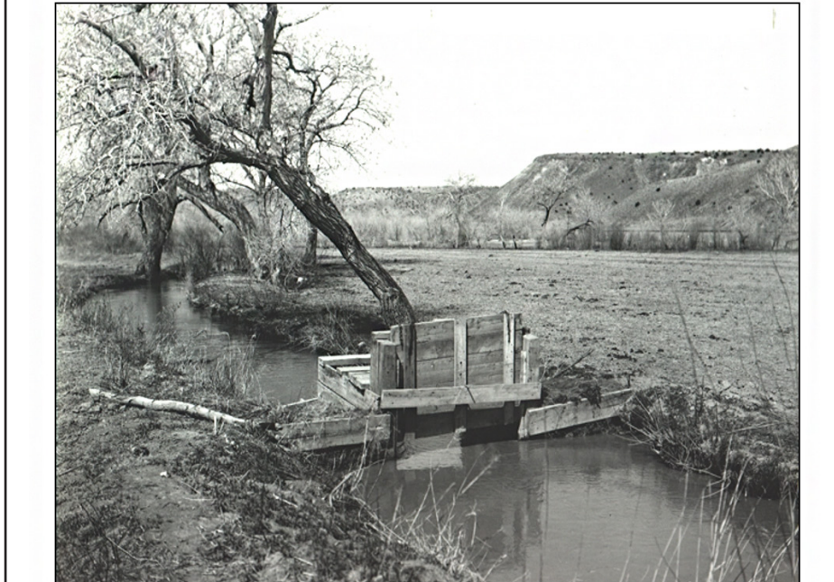
Figure 10. Middle Rio Grande Conservation District check structure at Algodones.
