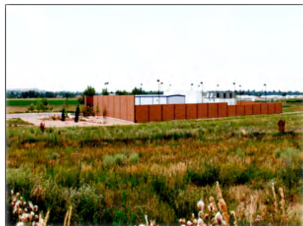
Figure 3. Completed Cloud Computing Facility in Longmont, Colorado
