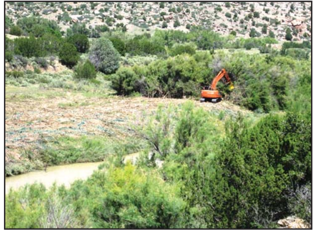
Figure 3. Mulching machine working on a 30-foot tall salt cedar
