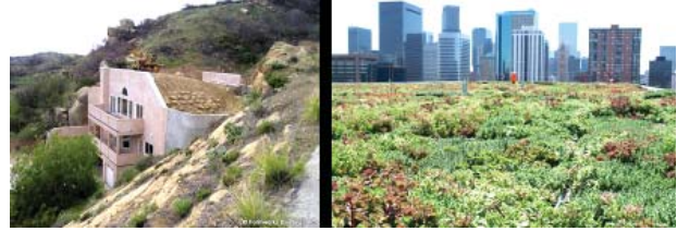
Figure 11. Green (ET) roofs
