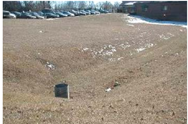
Figure 12. Infiltration basin leads water into a dry well
