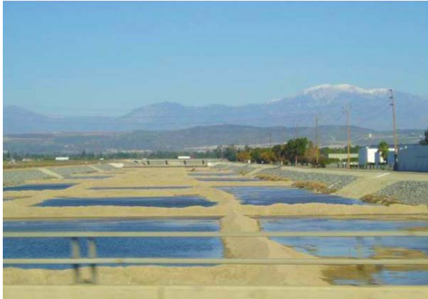
Figure 6. Artificial recharge project with levees on the Santa Ana River
