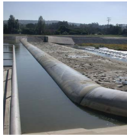
Figure 4. Inflatable dam diverting water from the Santa Ana River
