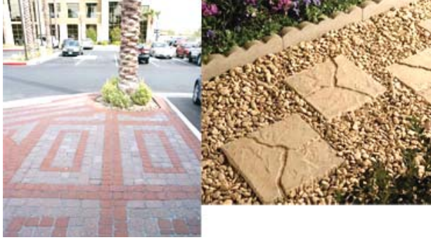
Figure 13. Permeable pavers promote recharge
