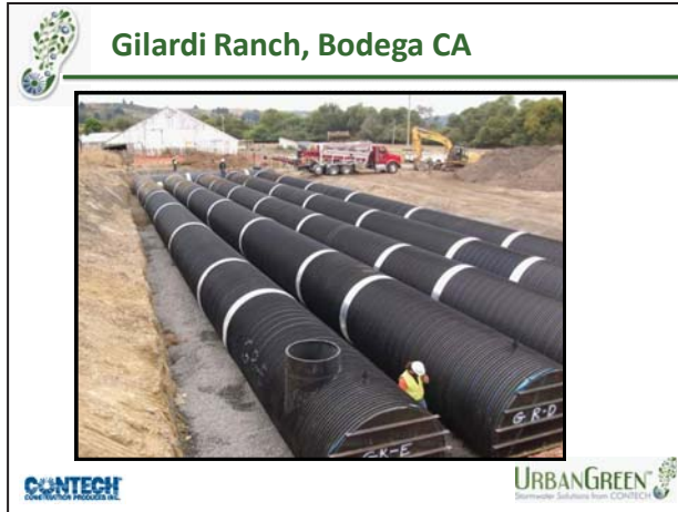
Figure 24. California ranch cistern system
