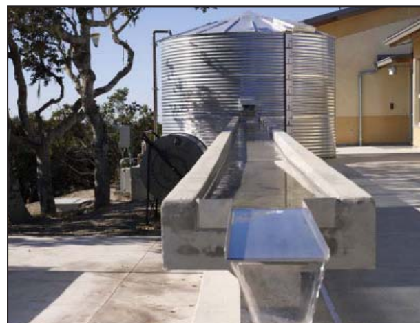
Figure 12. Passive rainwater harvesting design [Credit Sherwood Design Engineers]
