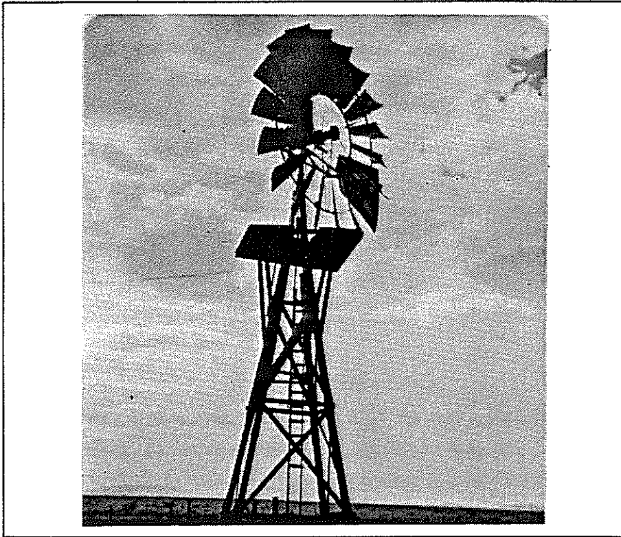
Figure 33. Camp Well #1, College Ranch. Windmill provided power to pump.
