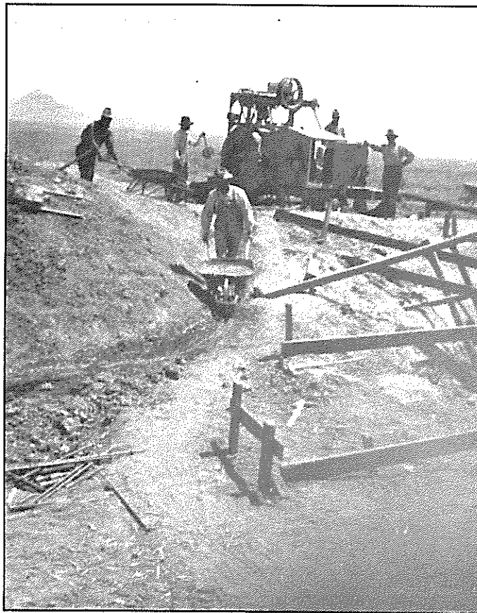
Cement mixer, East Side Canal, Dona Ana County. Photo courtesy of the Rio Grande Historical Collection, NMSU.
