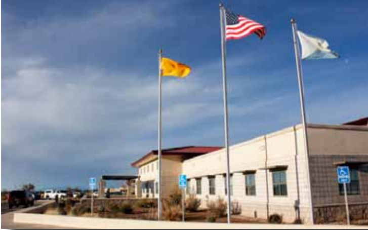
Most participants of the annual WRRI water conference attended tours of the Brackish Groundwater National Desalination Research Facility in Alamogordo.
