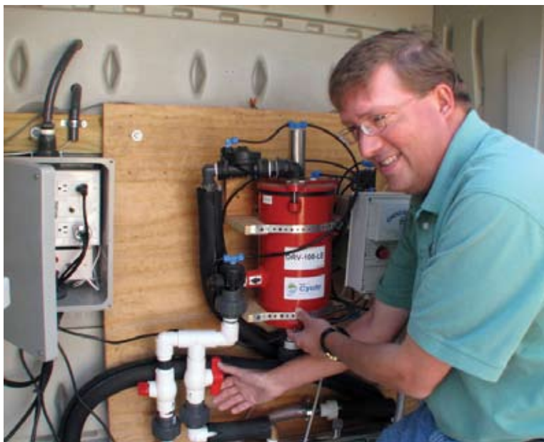
Turf scientist Ryan Goss checks a valve used to control sewage flow as part of an experiment to study the response of ornamental and turf grasses to water treated by a graywater system. About a dozen species will be tested and compared using treated graywater- and community-water irrigated plots at New Mexico State University.
